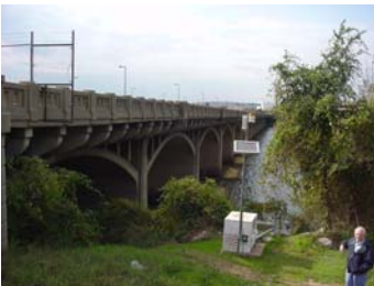
Old Route 66 Bridge
