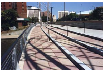
Example of pedestrian overlook on bridge – Wichita, Kansas
