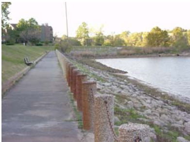
Pedestrian walkway adjacent to amphitheater/cove on west side of river
