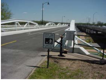
Jenks Pedestrian Bridge
