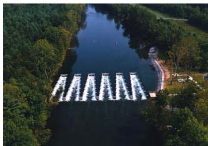
Labyrinth weir at South Holston Dam Tennessee Valley Authority
