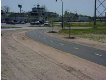
New trails adjacent to Aquarium Drive
