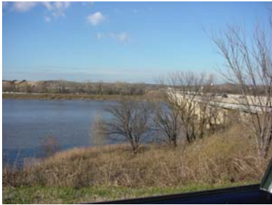
State Highway 97 Bridge / Arkansas River
