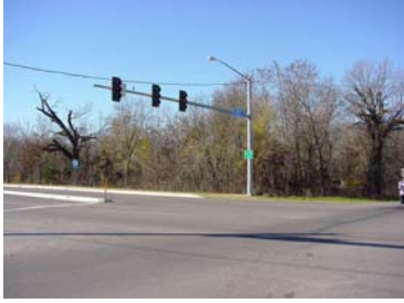
Newly signalized intersection at Aspen Ave. / Jasper Street
