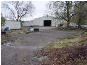
City of Broken Arrow maintenance facility (south of Aspen Avenue)
