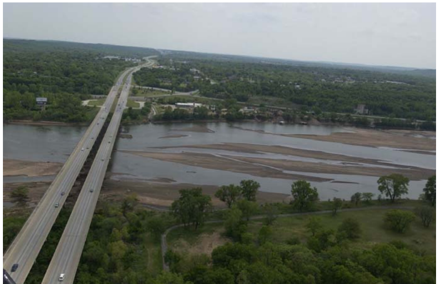
View south along Highway 97 Bridge in Sand Springs (Photo courtesy of Tulsa World)
