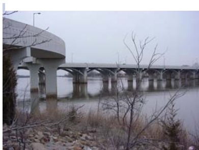
21 st Street Bridge
