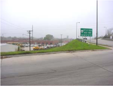
City of Tulsa maintenance facility (south of 23 rd Street.)
