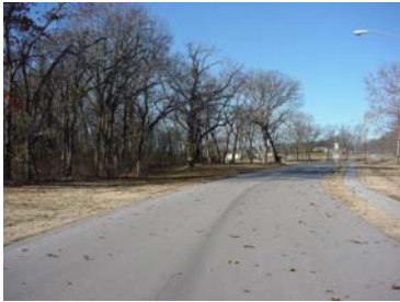
New park road through westside expansion area
