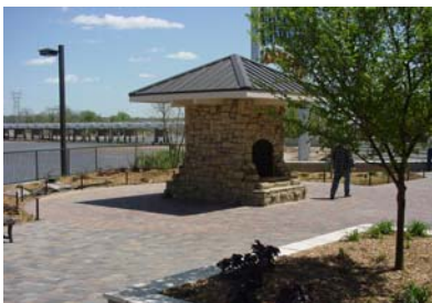
RiverWalk Crossing – outdoor fireplace
