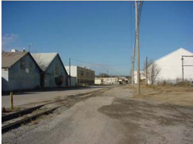
Industrial uses on S. Main Street.
