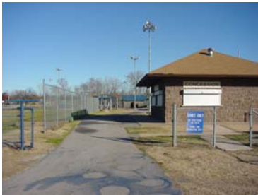
Typical Concession Building in Baseball Complex
