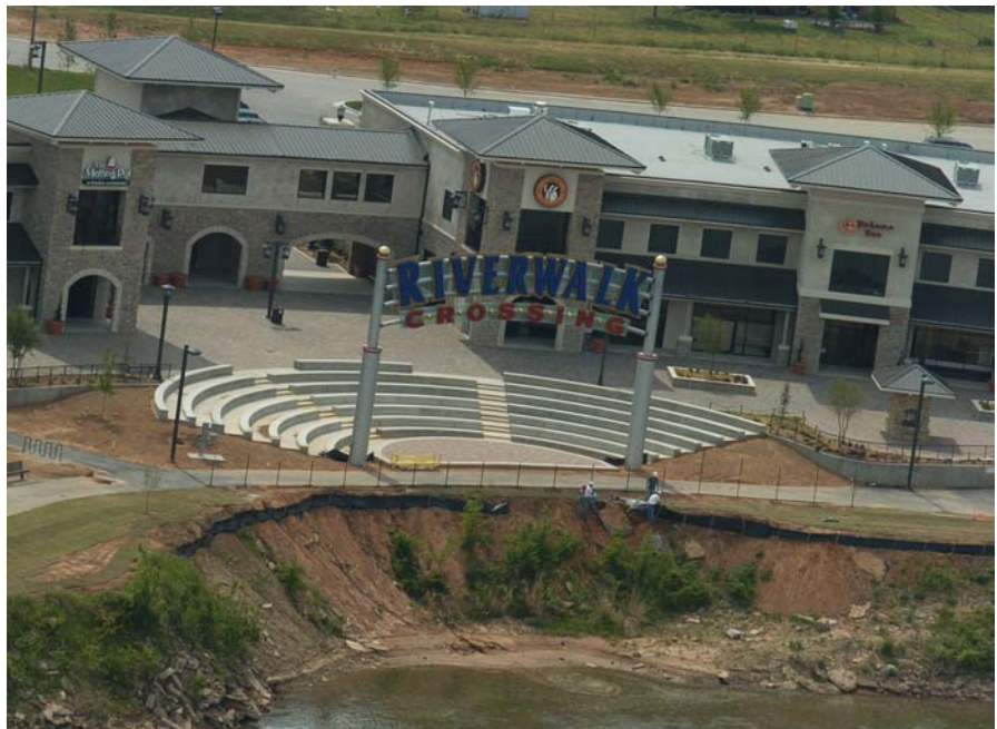
RiverWalk Crossing under construction (Photo courtesy of Tulsa World)
