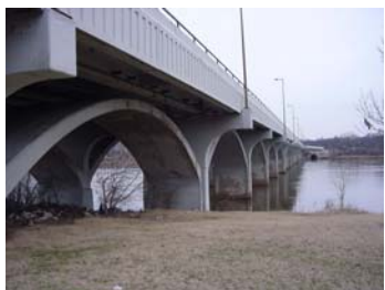
21 st Street Bridge
