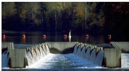
Close up of labyrinth weir at South Holston Dam
