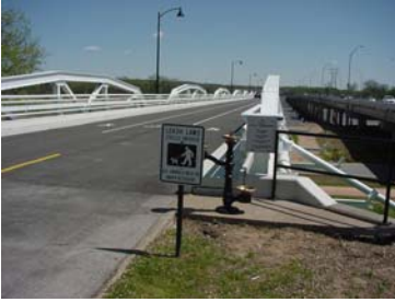
Jenks Pedestrian Bridge
