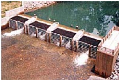
Infuser weir at Chatuge Dam Tennessee Valley Authority
