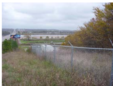
View looking east from bluff on south side of 71 st Street.
