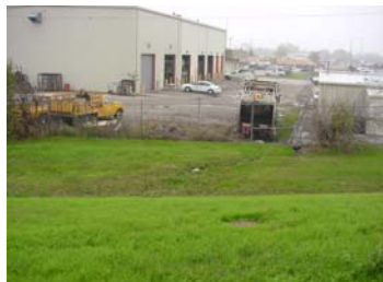
City of Tulsa West Yard facility
