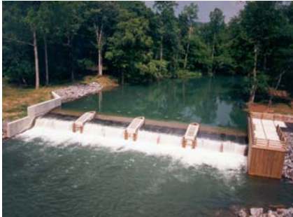
Infuser weir at Chatuge Dam Tennessee Valley Authority
