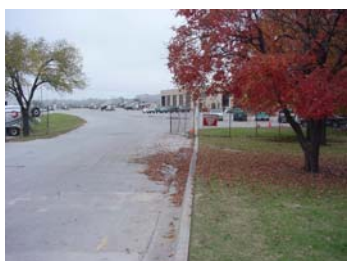
Concrete plant (north of 23 rd Street)
