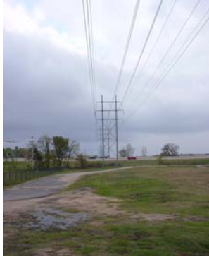
Overhead Electrical Lines
