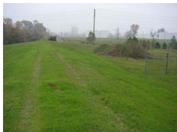
View along levee on west bank (south of 23 rd Street)
