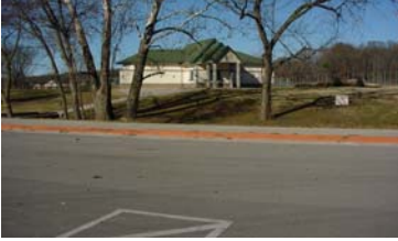
Concession / restroom facility in newest phase of Indian Springs Sports Complex
