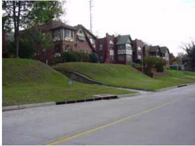
Architectural character (Riverside Drive – south of 11 th Street)
