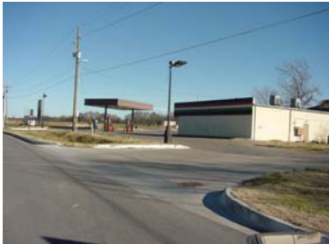
Convenience Store (Aspen Ave. / Jasper Street)
