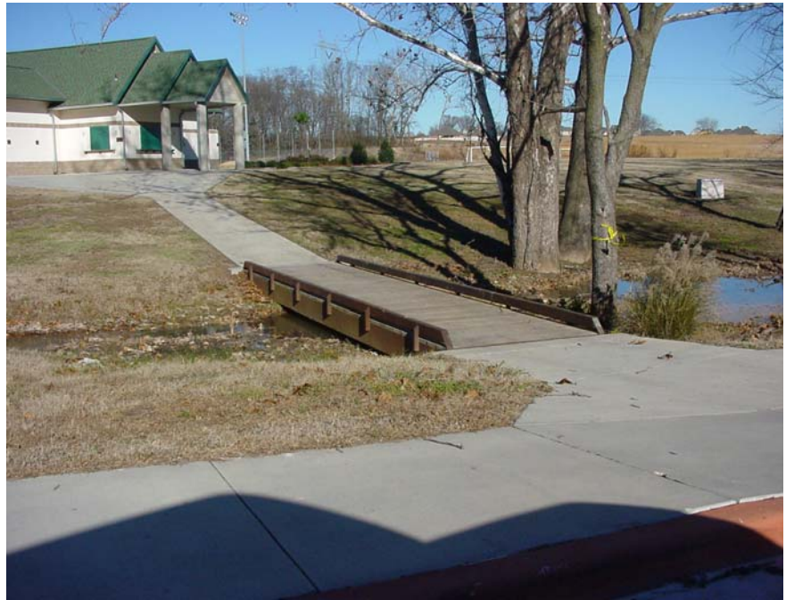
The new concession / restroom building at the west end of the park is accessed by a pedestrian bridge over a drainage swale.
