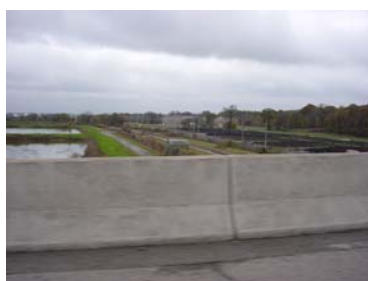
Sewage treatment facility on west bank (south of 71 st Street)
