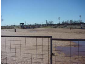
Existing rodeo arena
