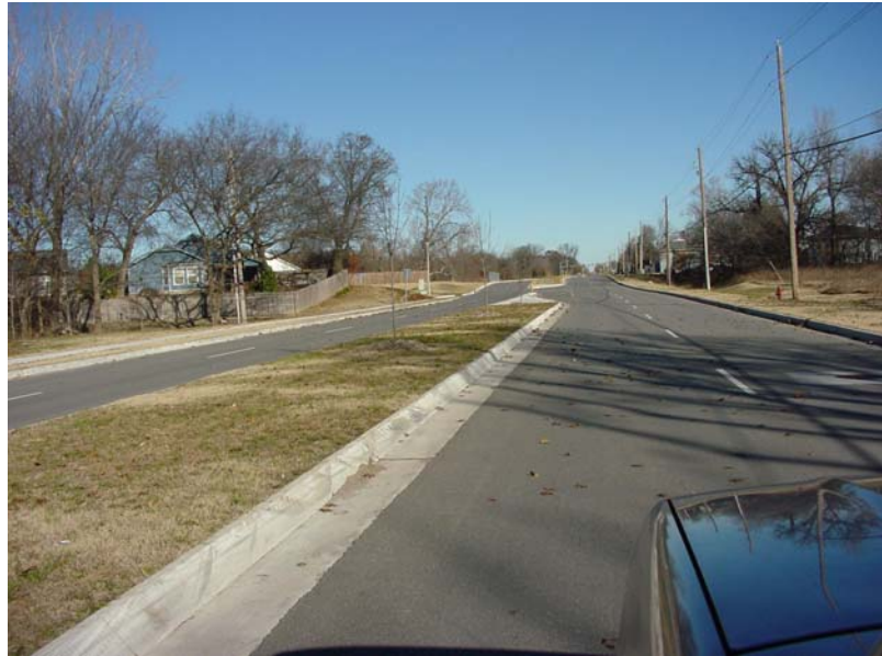
Aspen Avenue has recently been widened to four lanes, providing much better traffic movement to the sports complex.
