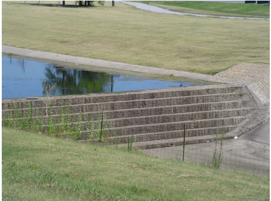
Example of a small stepped cascade weir on a drainage channel that flows into Mingo Creek in Tulsa,
