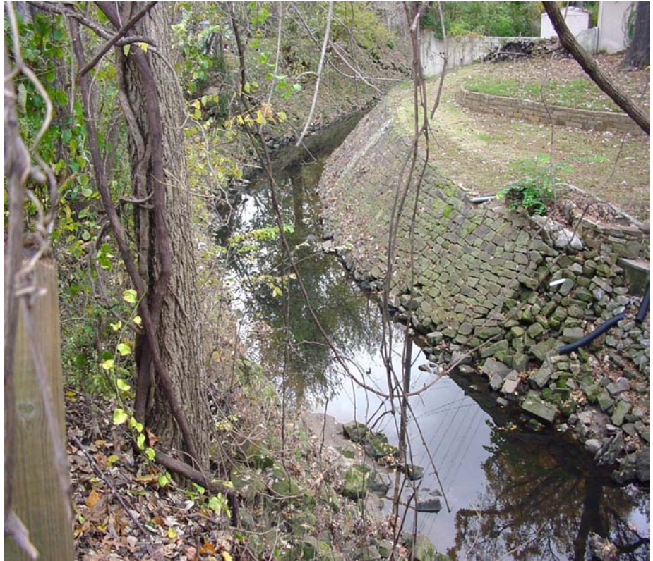
Existing stone lined bank along a portion of Crow Creek
