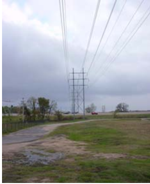
Overhead Electrical Lines
