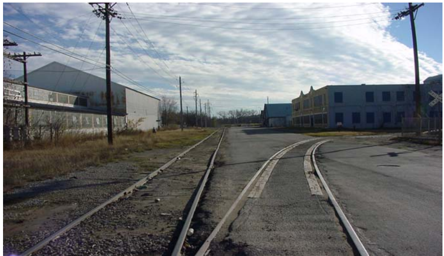
Active rail spurs along portions of Main Street will create a challenge to transforming the street into an attractive, pedestrian-friendly boulevard.
