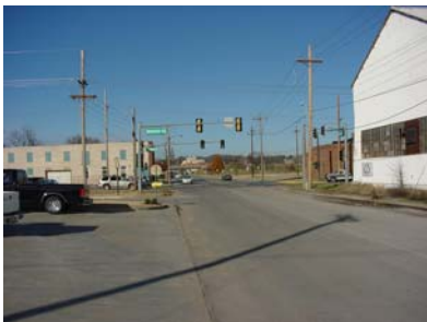
Intersection of Morrow Road / S. Main Street (view looking north)
